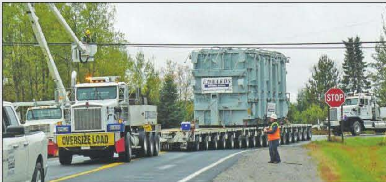
Crews work to truck a new transformer to the Arnold Substation in south Marquette County. The transformer is set to go online next year. (Photo courtesy of ATC)
